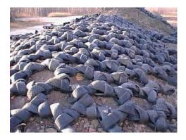
Mat: **starlike netting** Coverings (to be planted in holes) stabilization of slopes endagered to slip off
